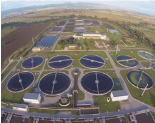
Kubratovo wastewater treatment plant
